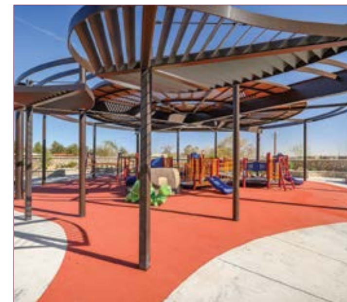
Exterior playground at the Youth Learning Center. The shade structure casts shadows consistent with Tigua art and patterns.
