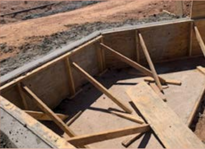
● The new construction of culverts designed to improve water runoff management.
