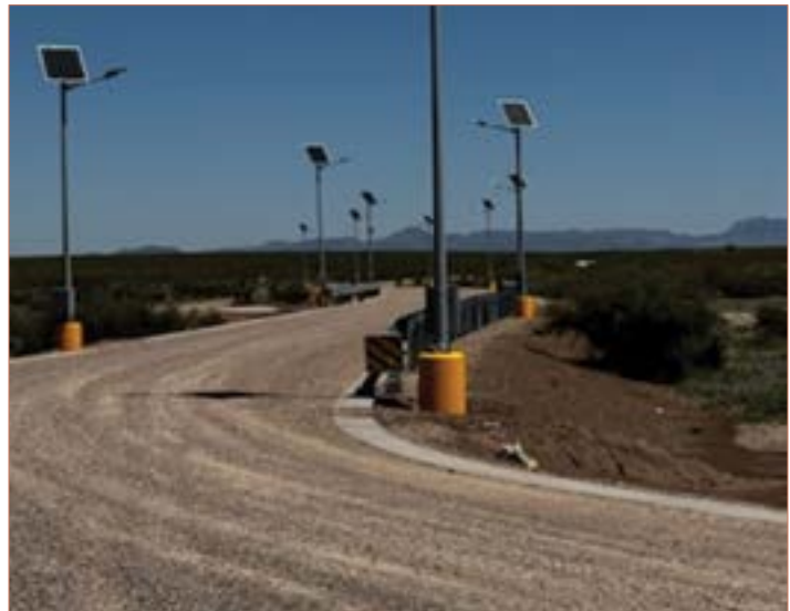
● Recent installation of solar lights to illuminate the Chilicote road
