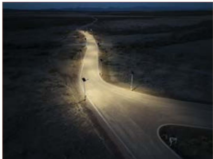
● The new Chilicote ranch bridge with additional lighting and road upgrades. This project was completed in 2024 and is the first of its kind for the Pueblo using Federal Highway money for bridge construction.
