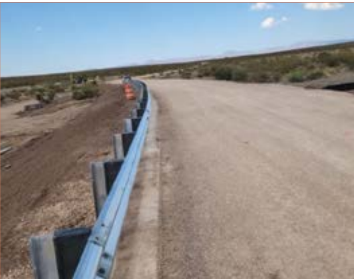
● New guardrails at the Chilicote Ranch.
